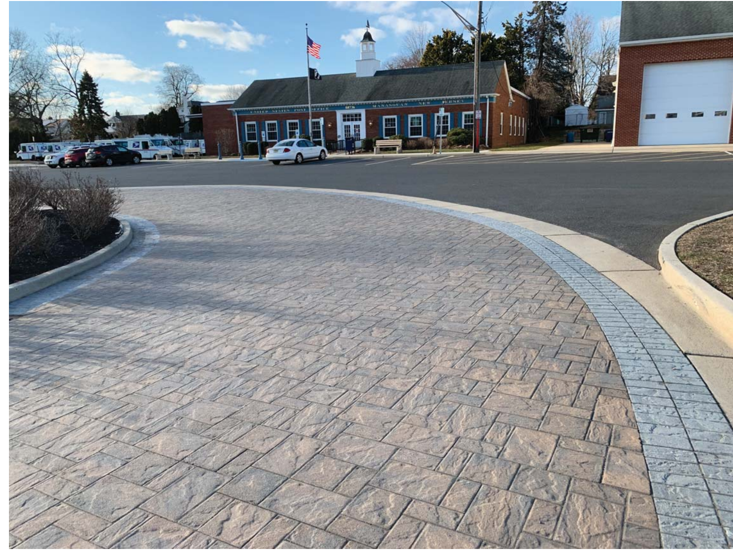
PAVING PATTERN (FROM ABE VOORHEES DRIVE)
